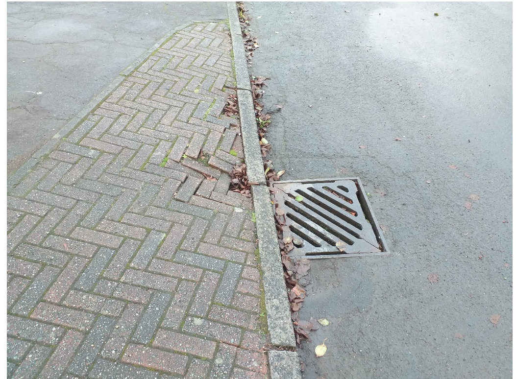
Front of [redacted] Sundrum Place: 2m2 sunken block paving in excess 20mm
